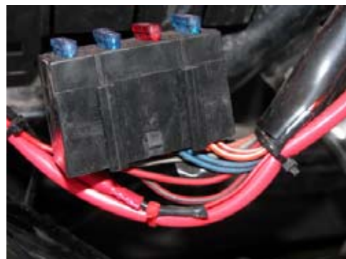
Alternative 12 volt from fuse box closeup
